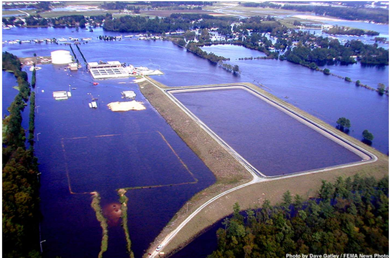
Greenville Utility Commission WTP after Hurricane Floyd, 1999
