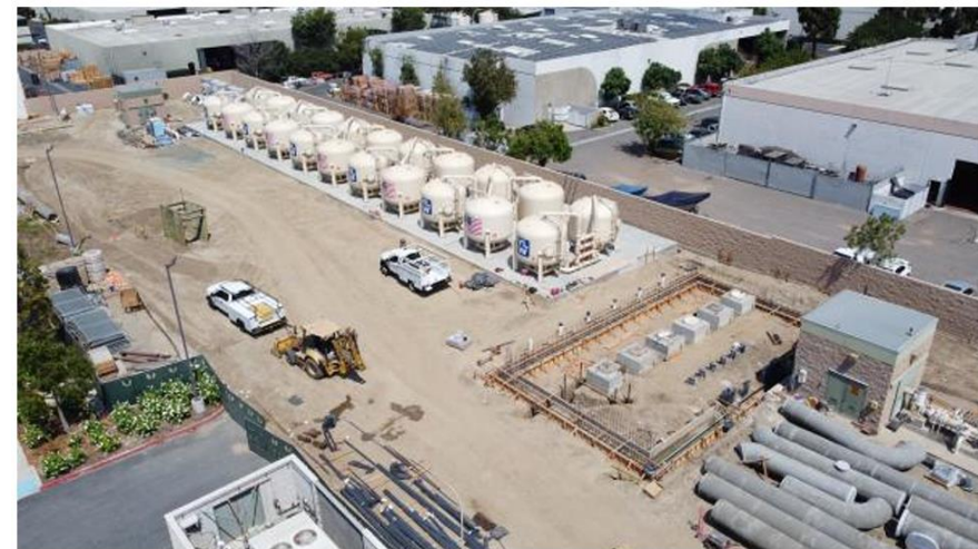
Photo credit: Orange County Water District
